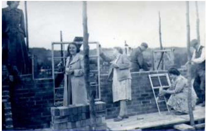
Painting the windows, July 1951
